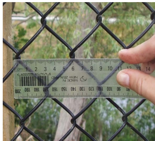
Figure 16. Mesh size on the predator (cat/dog) proof fence (6cm square)
